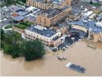
Floodwall protected Our Lady of Lourdes Hospital in Binghamton, Broome County, New York.
