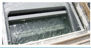
GROUND VENTS UNITS SIT BELOW STREET LEVEL GRATING TO PROTECT VAULTS, UNDERGROUND ROOMS AND SUBWAY STATIONS FROM FLASH FLOODING. DESIGNED WITH A WEEP HOLE TO MANAGE THE RATE OF WATER ENTERING THE UNDERGROUND SPACES, THE SYSTEM PREVENTS THE OVERPOWERING OF PUMP STATIONS.
