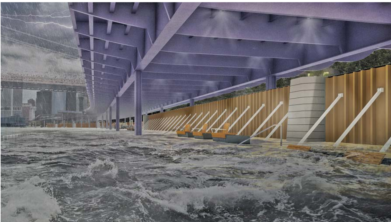
Flip-up gates, which are activated in extreme storms, are designed to lay flat in normal weather conditions. Renderings courtesy of NYC DDC
